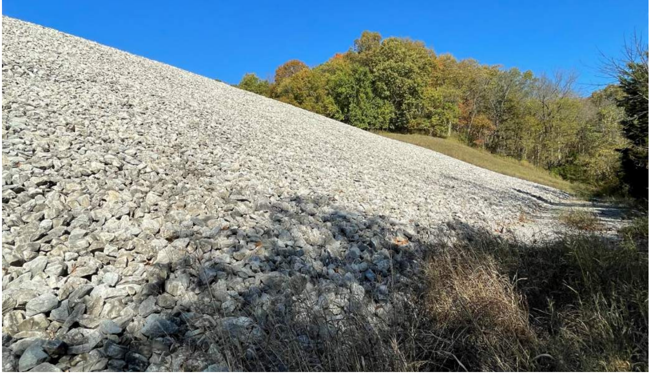
Photograph 14 – Downstream side of dam, previous rip rap slope. Looking east.
