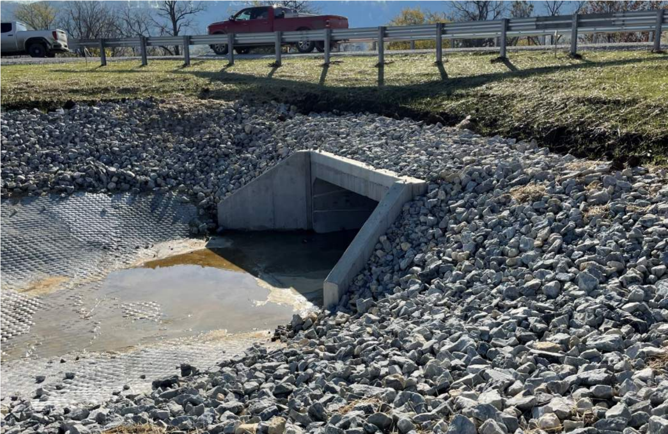
Photograph 17 – Upstream side of dam at new 12x4 culvert.
