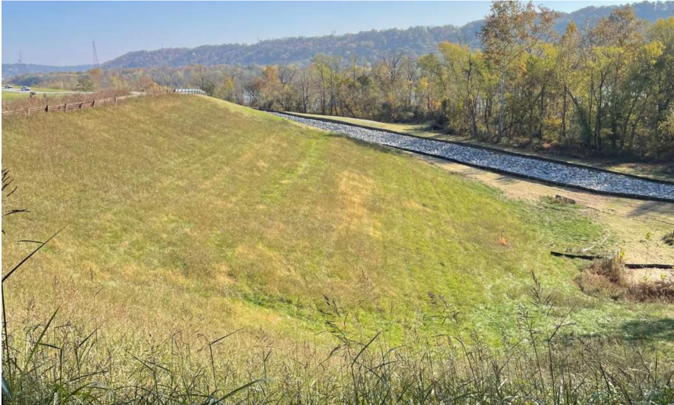
Photograph 1 – West downstream side of LRCP looking east.
