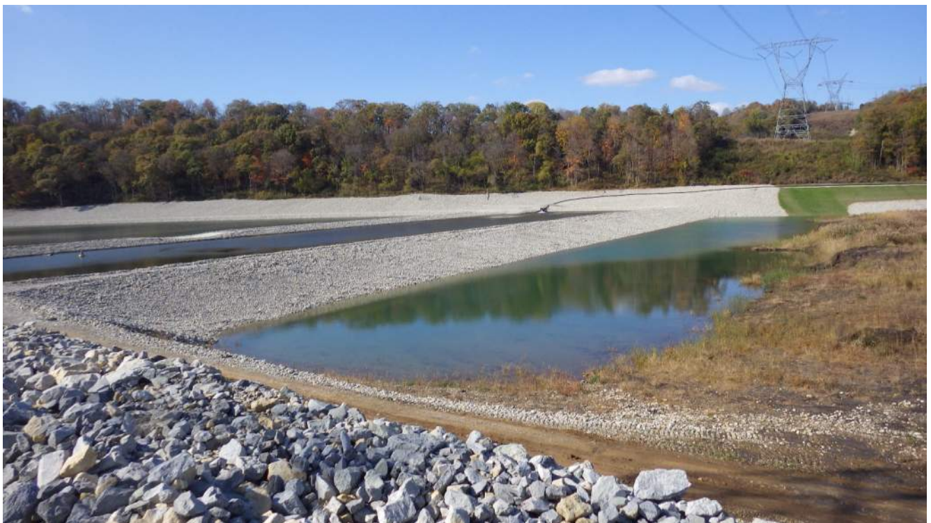
Photograph 12 – Looking north and west across western settling ponds from the southern dike embankment.
