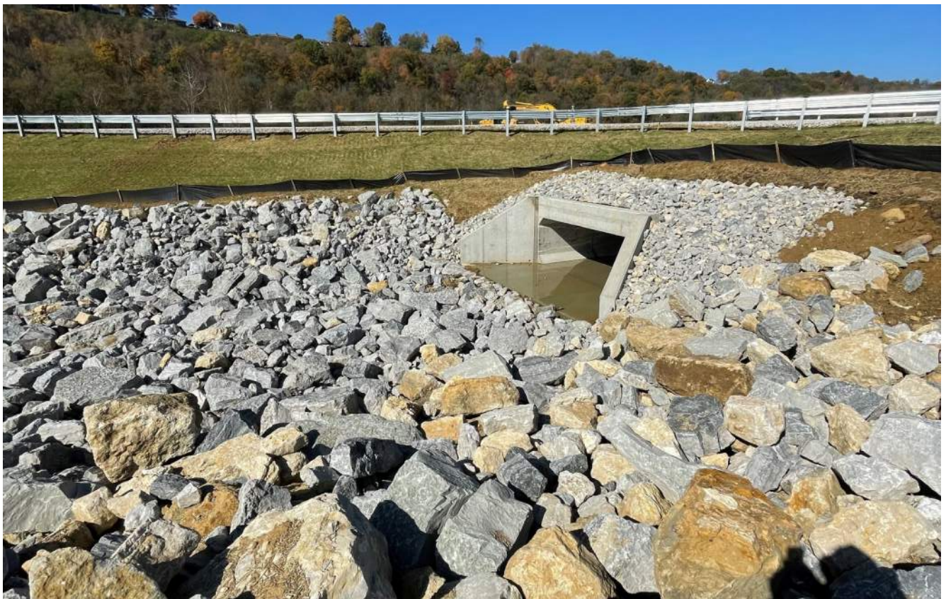
Photograph 19 – Downstream side of dam at new 12x4 culvert.
