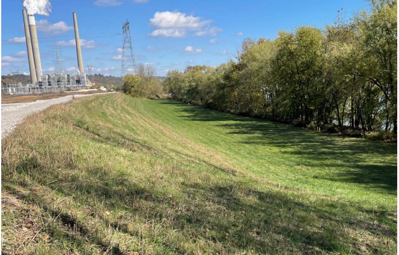
Photograph 5 – South dike embankment, downstream side looking east.
