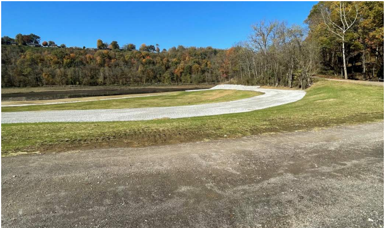
Photograph 15 – Crest of dam at the east end, looking north at new access road and teardrop area.
