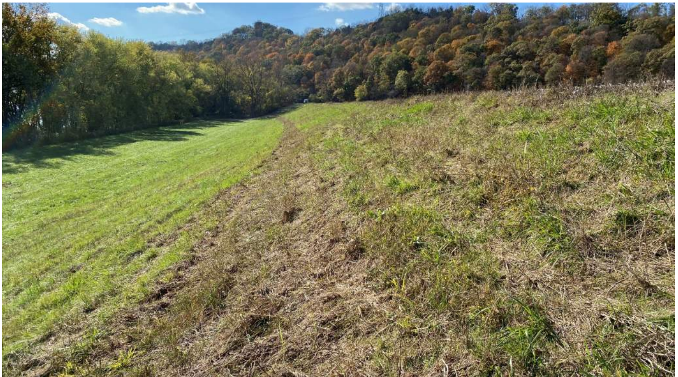
Photograph 10 – Southern dike embankment downstream side, showing damaged vegetation from vehicle traversing slope.
