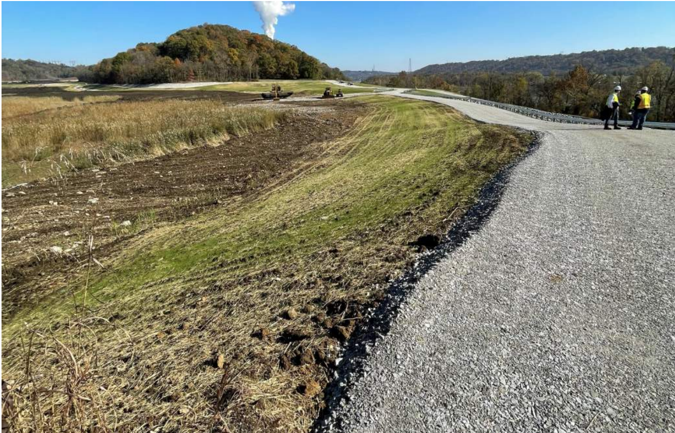
Photograph 2 – West upstream side of LRCP looking east. Starting from recent construction.
