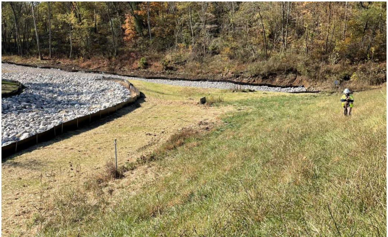
Photograph 4 – Western downstream side of dam where new channel area and toe meet.
