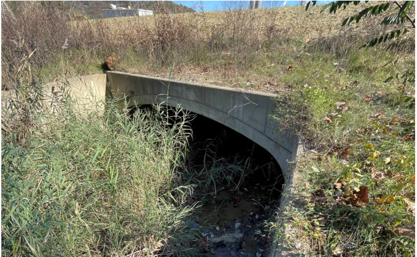
Photograph 1 – Northwest (upstream) side of inlet culvert structure, northwest side of WBSP
