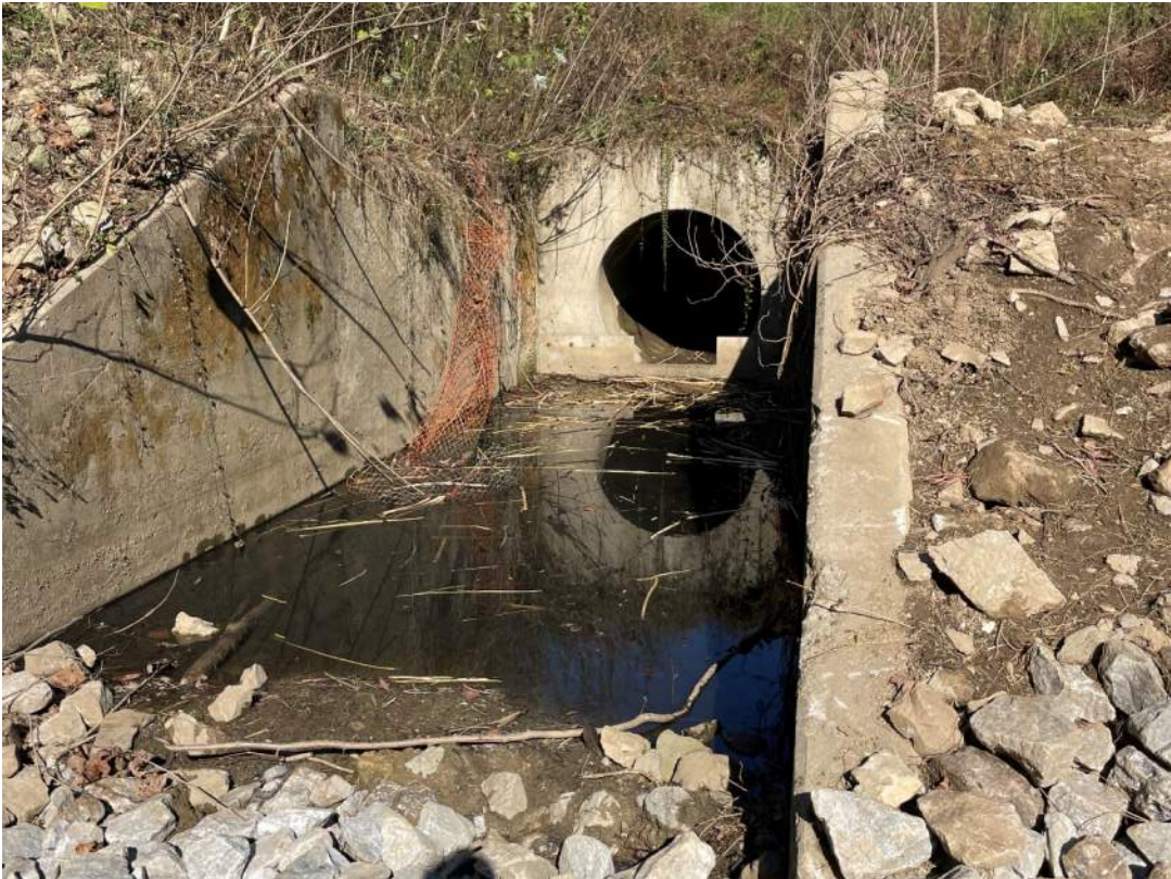
Photograph 5 – Outfall 001 outlet structure at toe of dam.
