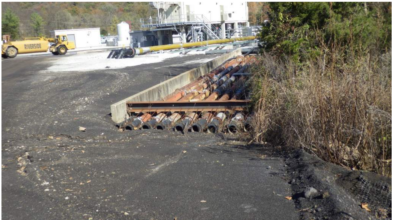
Photograph 2 – Former CCR sluice pipes, terminated, northeast side of WBSP.
