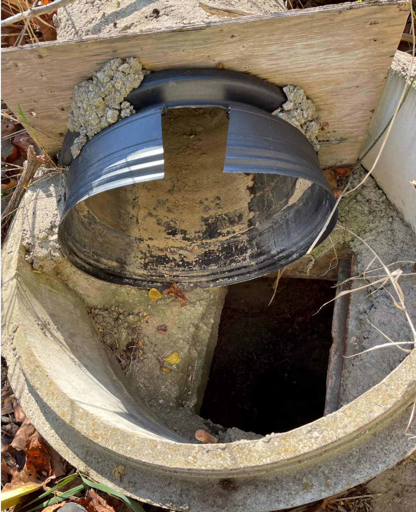
Photograph 8 – Current inlet structure for Outfall 001.
