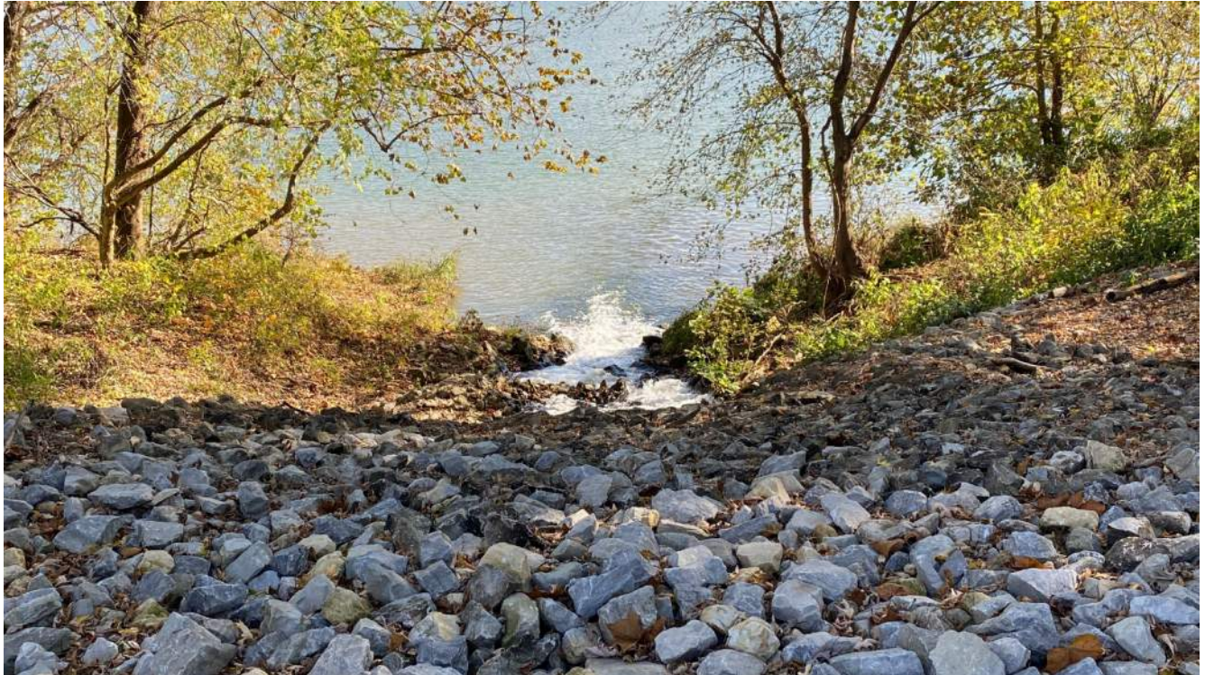
Photograph 9 – WBSP Outfall outlet to the Ohio River.
