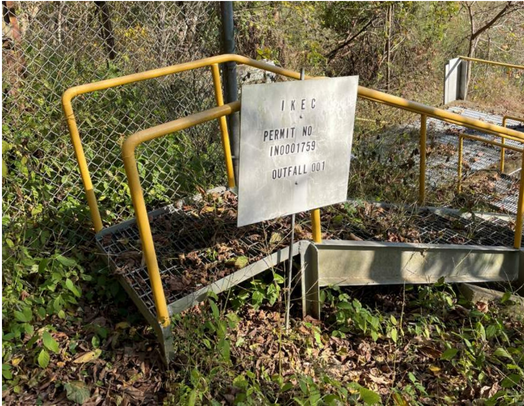
Photograph 6 – Access to inlet of Outfall 001.
